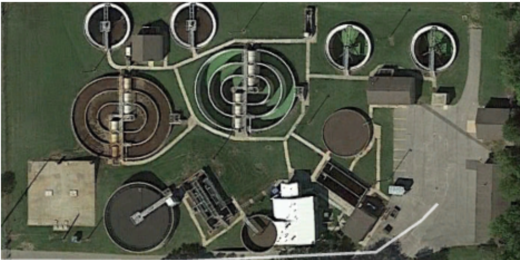
Mechanical Treatment Overview
