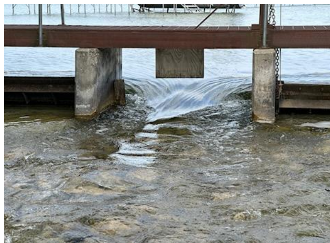
Cut River Dam September 25, 2023
