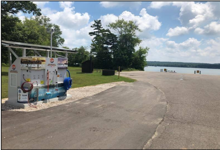
Figure 44. A public boat washing station at North Higgins Lake State Park.
