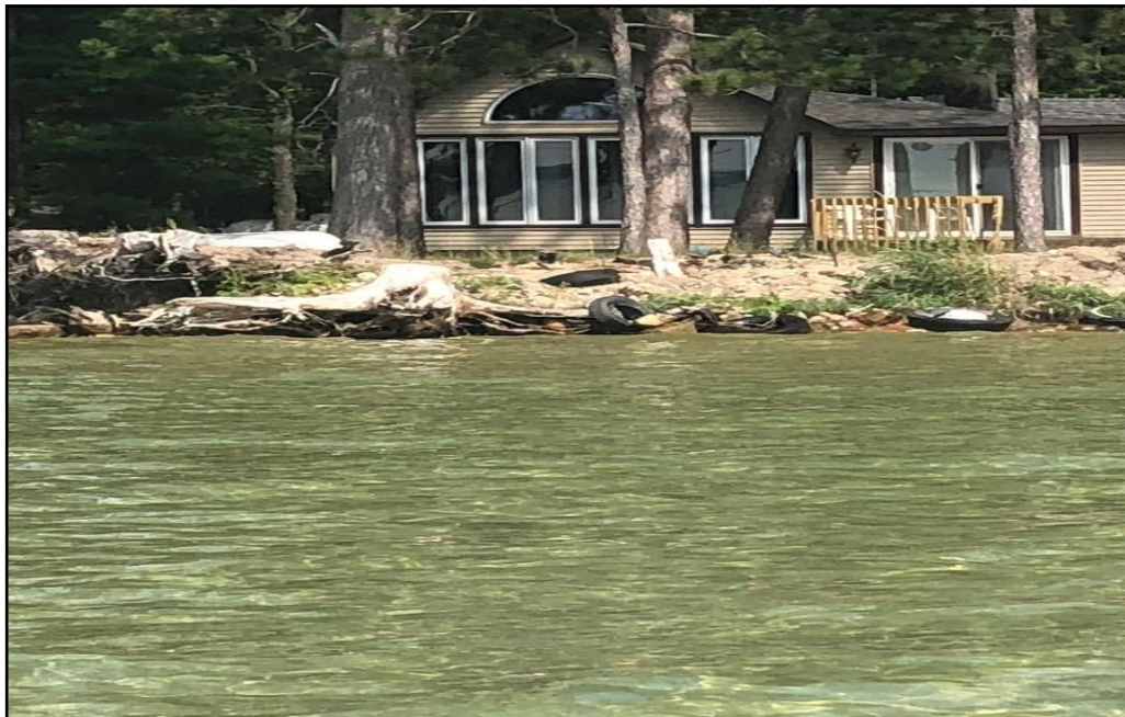
Figure 61. Higgins Lake shoreline erosion (August 21-23, 2019).
