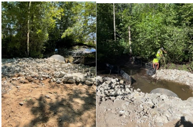
After Culvert Replacement Photos
