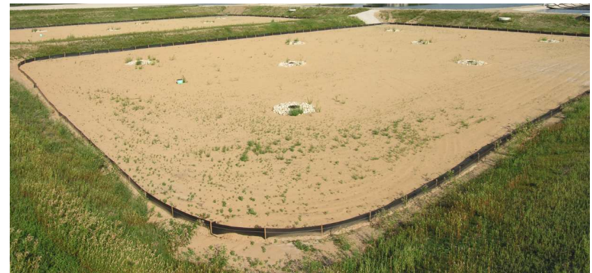
Rapid Infiltration Basin
