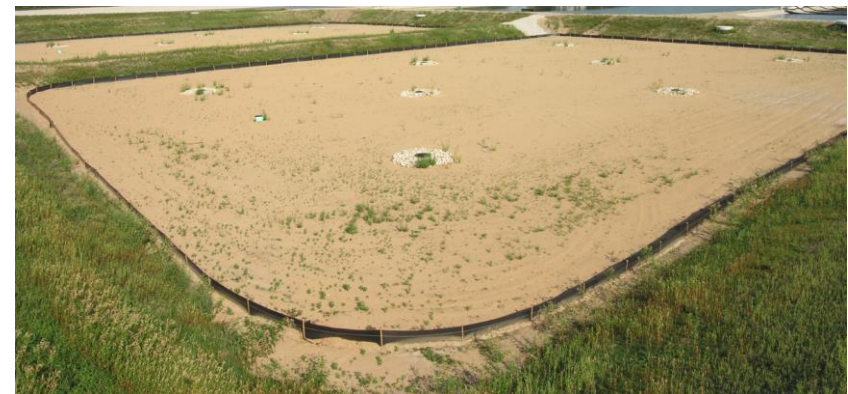
Rapid Infiltration Basin
