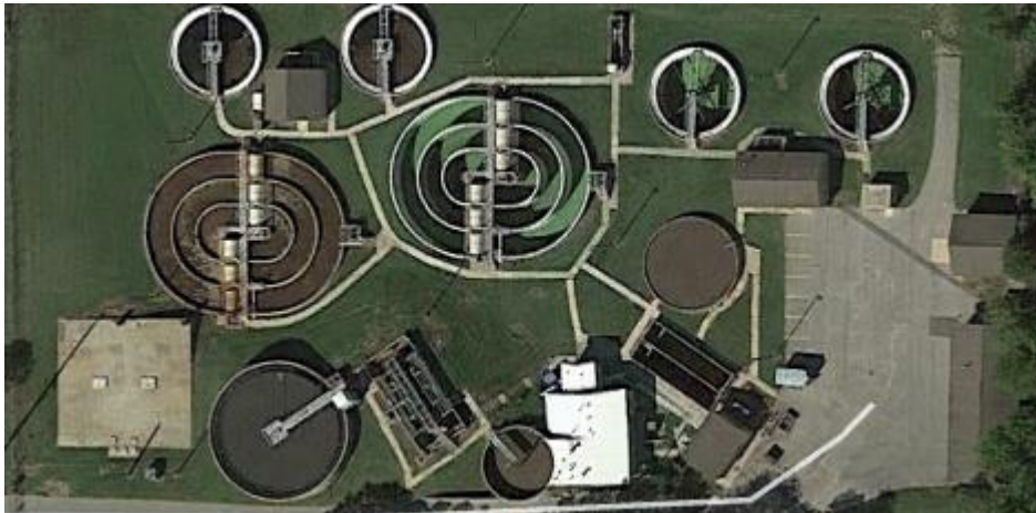
Mechanical Treatment Overview
