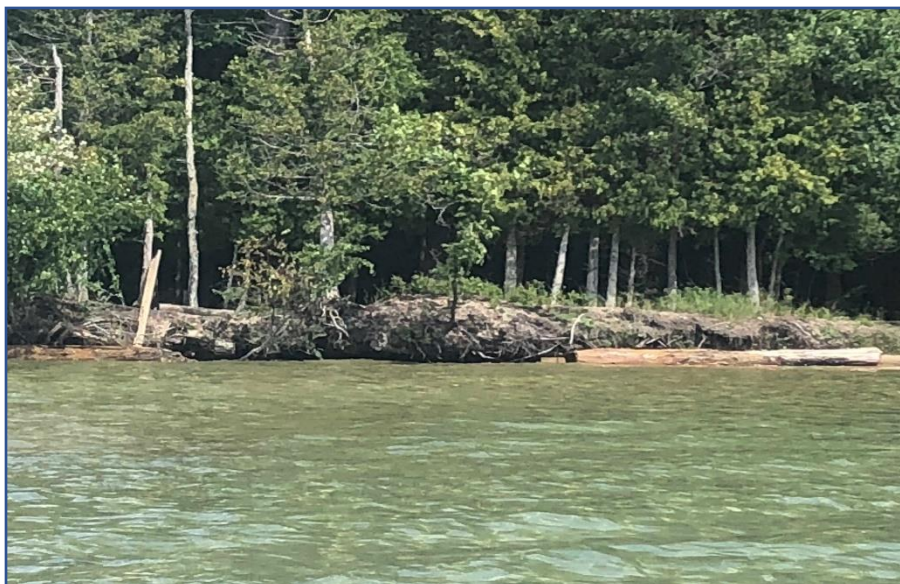
Figure 60. Shoreline erosion on Higgin Lake with bank undercutting (August 21-23, 2019).
