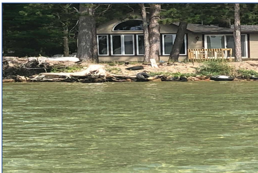
Figure 61. Shoreline erosion around Higgins Lake (August 21-23, 2019).
