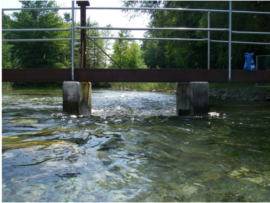
Unregulated span viewed from upstream face.
