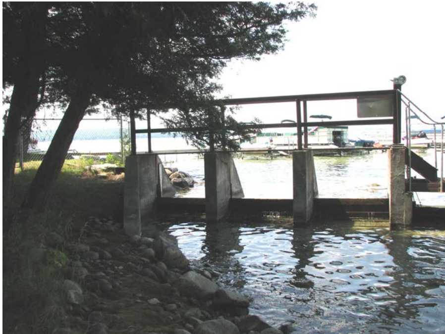
Downstream face of three stop log bays.
