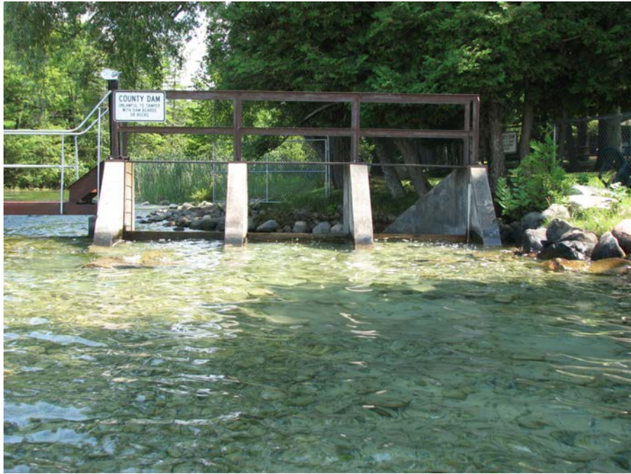
Upstream face of three stop log bays.
