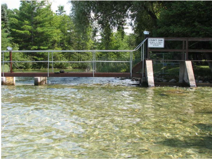
Upstream face of southernmost flopp gate.
