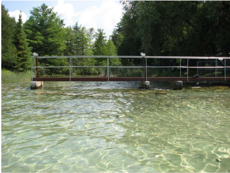
Upstream face of center flop gate.
