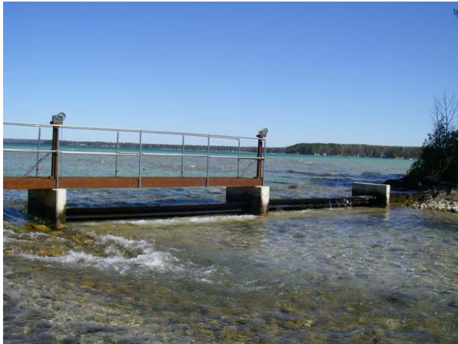
Downstream face of center (left) and northern flopp (right) gates.
