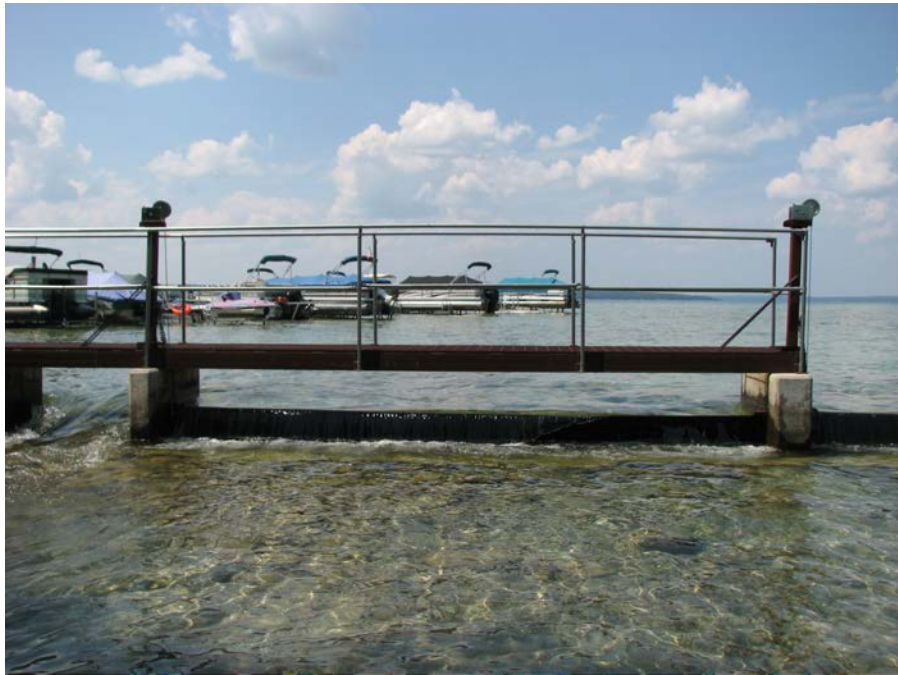
Downstream face of center flop gate.
