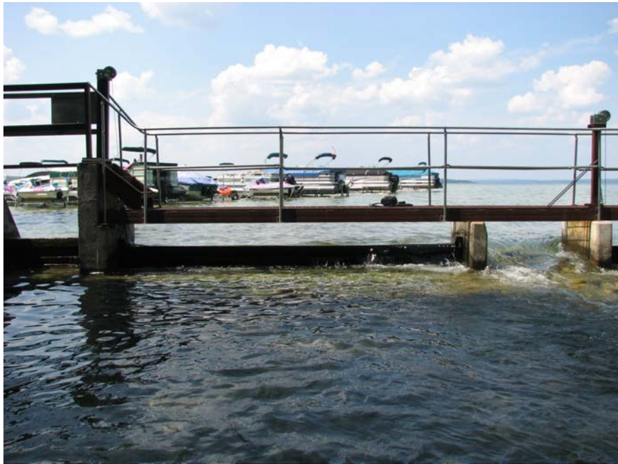
Downstream face of southernmost flopp gate.
