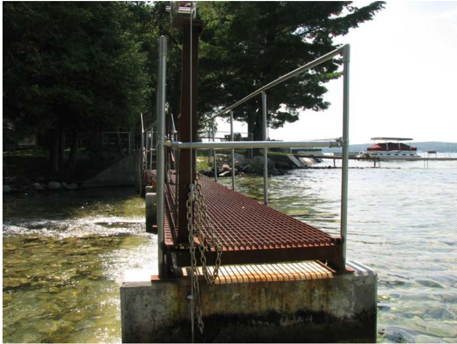
North end of decking/railing.
