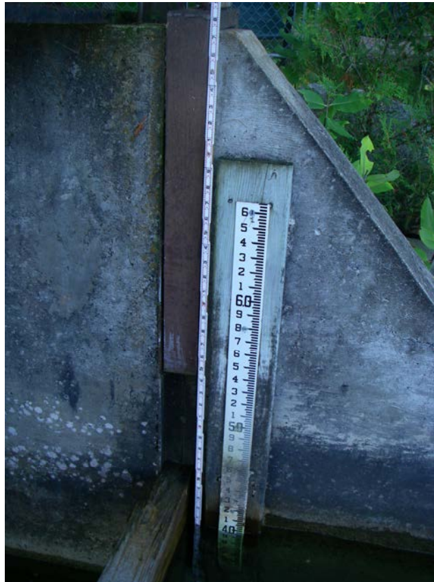
Staff gage on southernmost pier of southern stop log bay.
